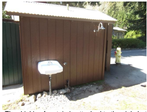
The drinking fountain is attached to the sink, but turns on separately.
