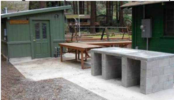
New sink with Virgil's kitchen in background.
